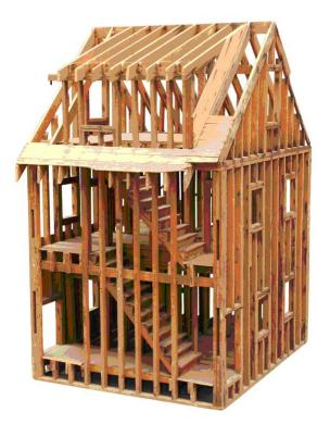
Balloon framing construction detail. This method of building made construction quicker – using prefabricated elements (such as studs and joists). It is easily identifiable by two story studs and was common through the nineteenth century.
