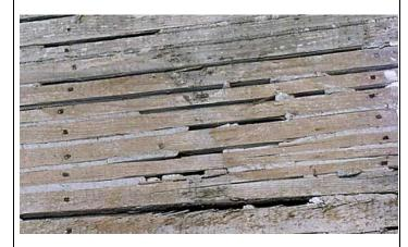
Split lathe wall with plaster removed. Individual boards are nailed to the stud then plaster is applied over. Usually studs and lathe were not level and the professional plaster ensured level walls.
